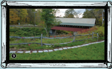
Established and kept up by the Brattleboro Garden Club, the Creamery Bridge Park Gardens serve both as a peaceful setting and an affirmation of the beauty of the old covered bridge and its historic importance.
